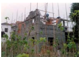
11. Pulling off the 1 st floor
