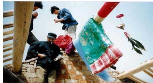
6. Putting up roof tree
