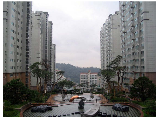
Fig. 5. View of 'New' Nangok upon completion of redevelopment.
