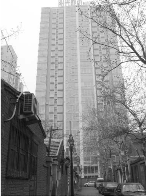
Figure 1. A high-rise block of flats in Sun City estate, Xinzhongjie, Beijing
