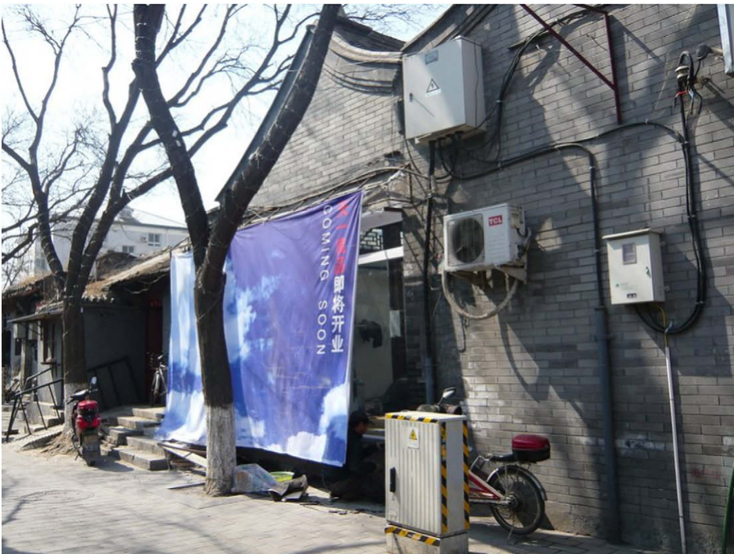
Fig. 4. A new shop under refurbishment. © Hyun Bang Shin, March 2009.
